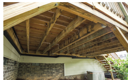
Decks, awnings, eaves offer protected roosting areas for mosquitoes
